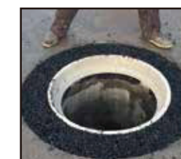
3.After Breaking & Filling
